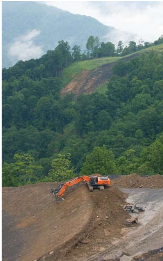
Smaller Hitachi excavators are used for reclamation.
