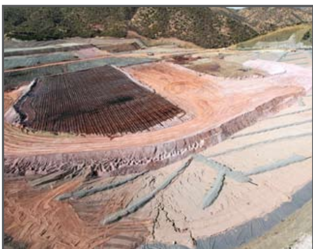
The leach pad is double-lined and monitored for leakage.
